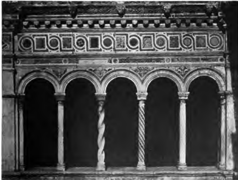
DETAIL OF A ROMANESQUE ARCADE Architecture enriched with a Byzantine treatment of mosaic. The carving and the diversity of the columns also show marked Byzantine characteristics (Cloister arches of St. Paul-Beyond-the-Walls, Rome)
